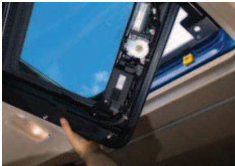
Preparation: removal of the existing roof window
