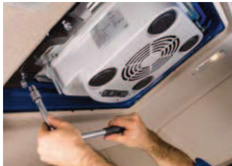
Fits like a custom-made unit: the CA 800 replaces the roof window
